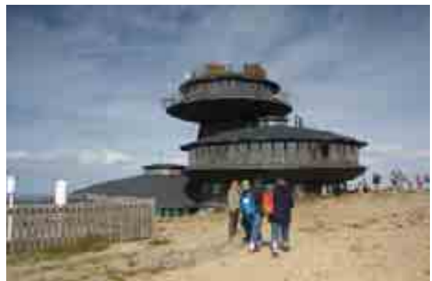
Fig. 5. The observatory on Śnieżka – present condition
