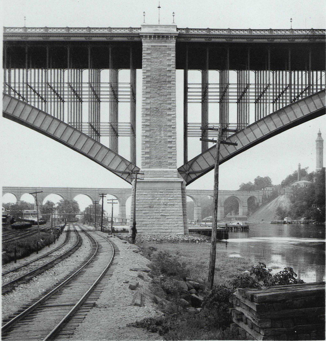
CENTRAL PIER, WASHINGTON BRIDGE.
