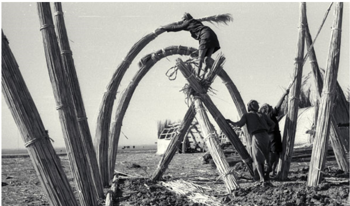
Fig. 2.2 Bending the bundles bufixed at the ends to the ground and tying them together at the top. 8
