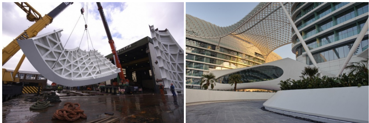
Fig. 2.11 Link bridge in Yas Marina Hotel. Left: in CIG shipyard 28 , right: completed structure 29 .
