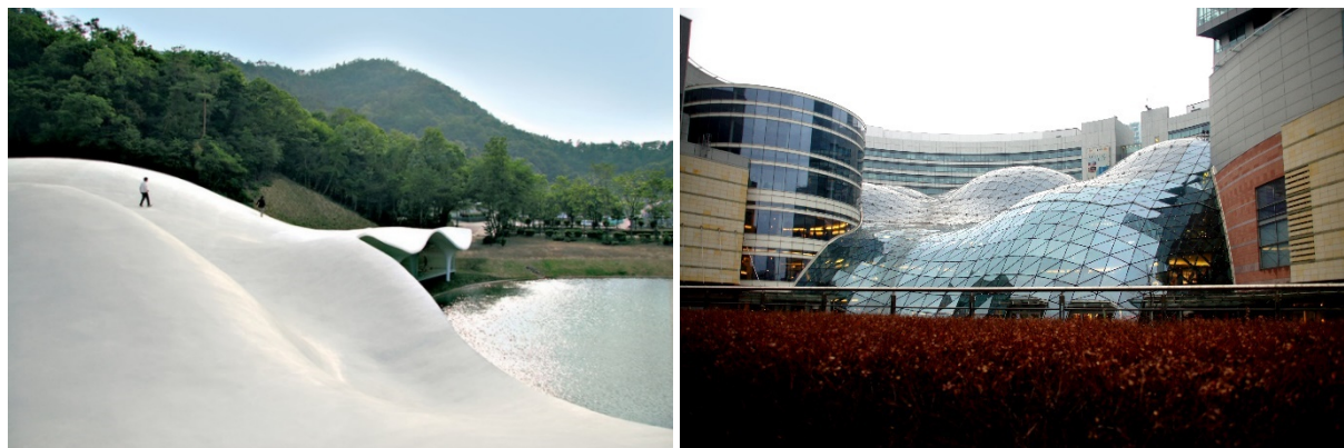
Fig. 3.2 Left: continuously curved shell (Crematorium in Kakamigahara) 39 , right: discrete lattice shell (Złote Tarasy, Warszawa) 40 .
