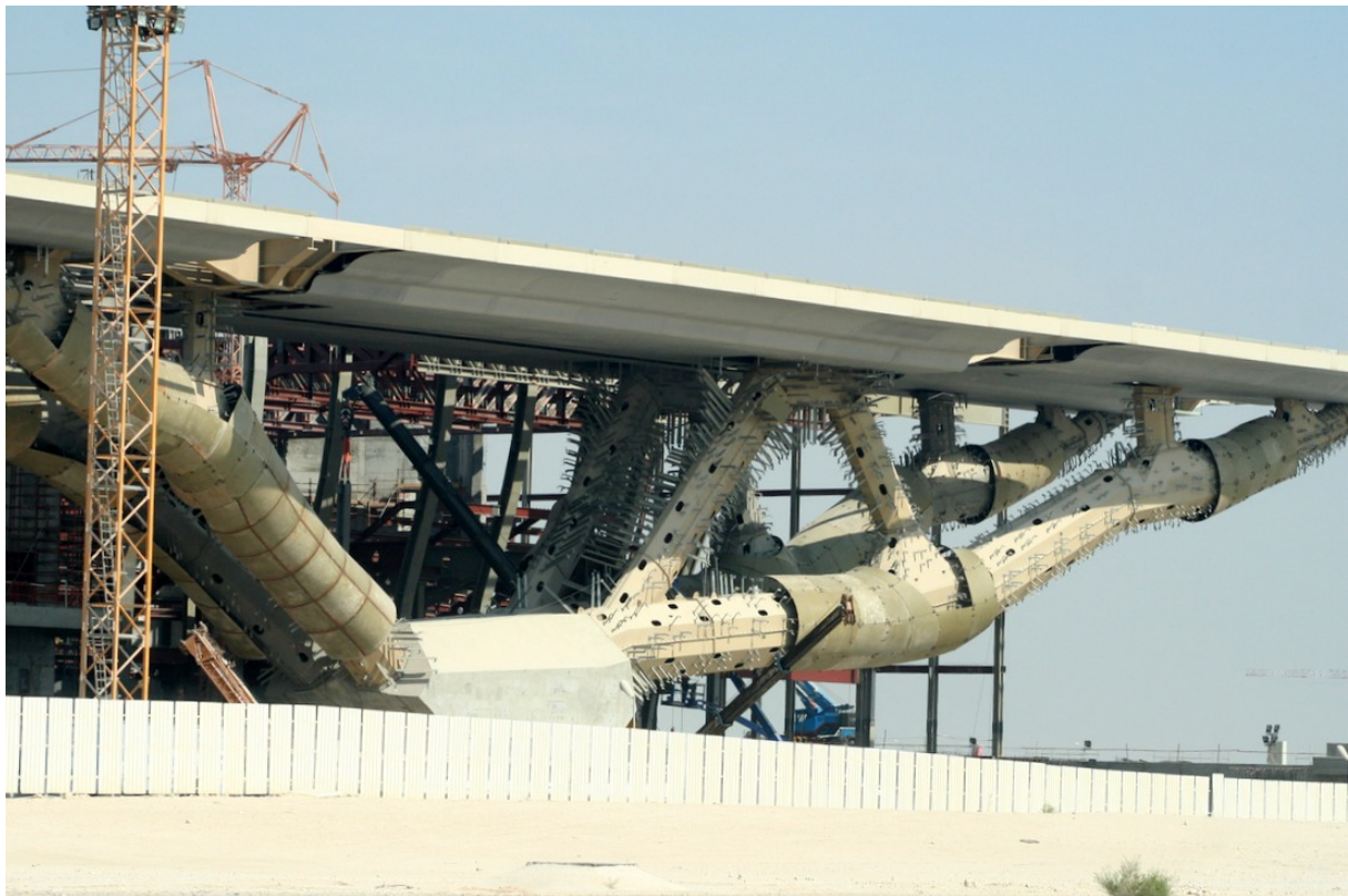
Fig. 3.1 Tree-like structure at Qatar National Convention Centre. Internal, octagonal structure made of planar steel plates partially covered by freeform cladding. 35
