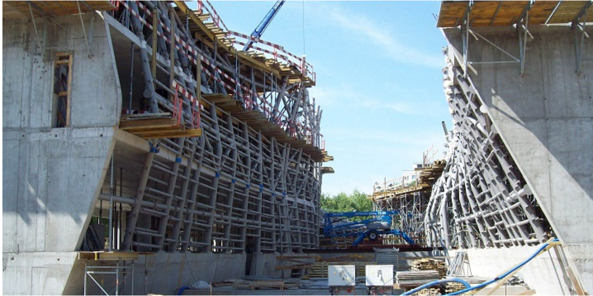
Fig. 2.12 Steel structure behind the freeform walls. 32
