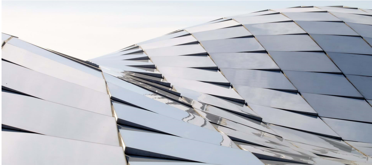
Fig. 3.3 Planar, quadrilateral glass panels with non-collinear adjacent edges. Kogod Courtyard glazed roof, Smithsonian Institution, Foster + Partners. 42
