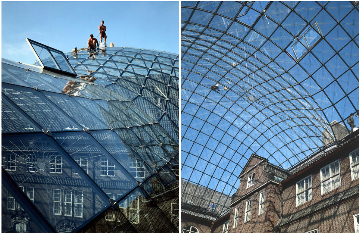
Fig. 4.9 The glazed canopy over the courtyard of Museum of Hamburg History - an example of translational PQ grid shell. 55
