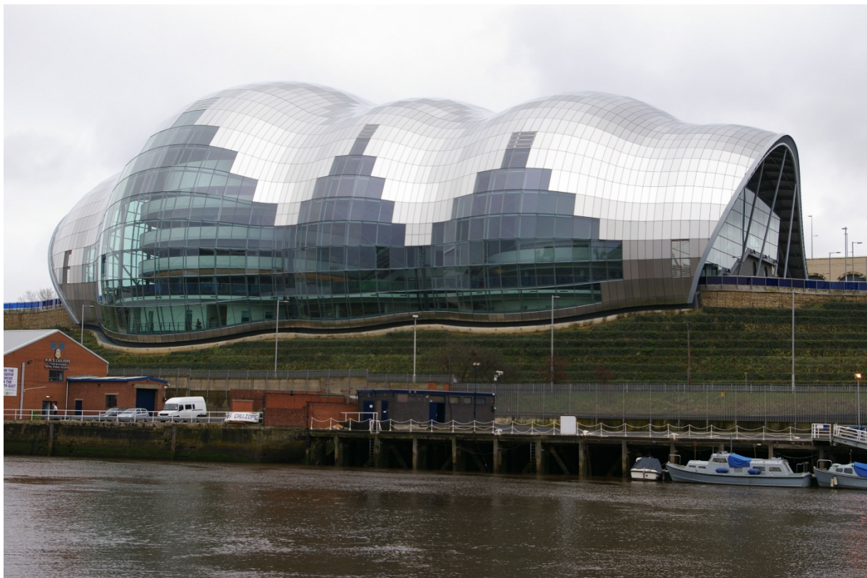
Fig. 4.23 Sage Gateshead - architecture: Foster + Partners. An example of scalar - translational PQ mesh. 59
