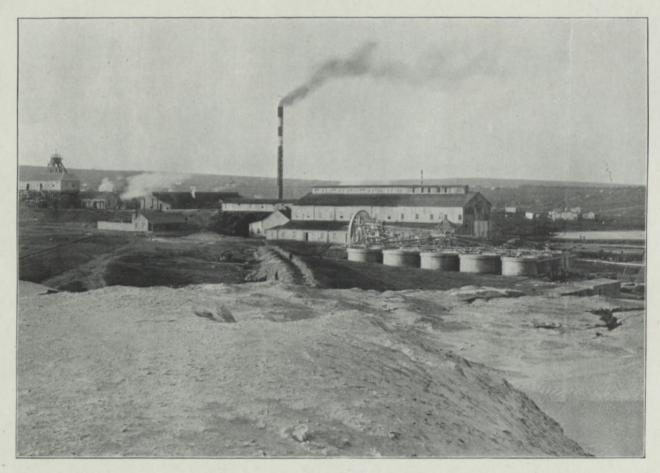
PLATE II.-HEADGEAR, SORTING-HOUSE, MILL-HOUSE, TAILINGS WHEEL, AND COLLECTING VATS, NEW PRIMROSE MINE.
