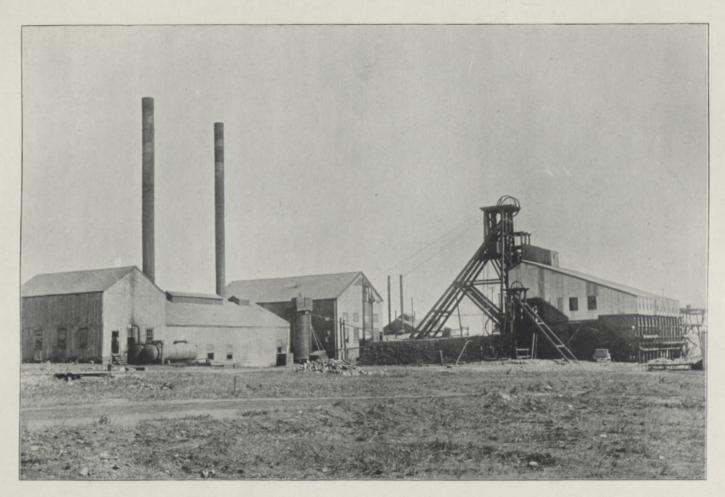
PLATE VI.-HEADGEAR (VERTICAL SHAFT) AND ENGINE-HOUSE, FERREIRA MINE.
