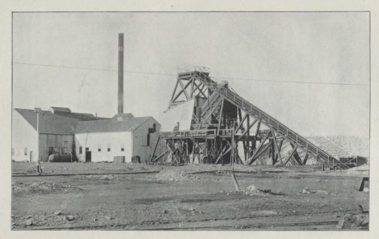
PLATE XIII.—HEADGEAR (INCLINED SHAFT) AND ENGINE-HOUSE, GELDENHUIS ESTATE MINE.
