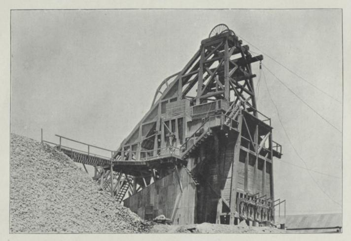
PLATE VII.-HEADGEAR (INCLINED SHAFT), ROBINSON MINE.
