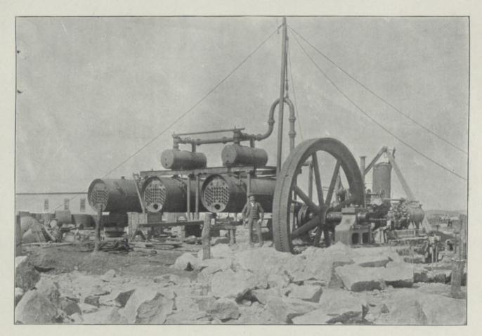
PLATE IX.-BOILERS AND ENGINE IN COURSE OF ERECTION AT THE WOLHUTER MINE.
