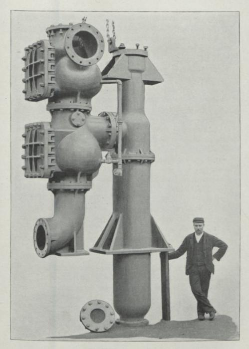
PLATE XI.—CORNISH PUMP. Diameter of ram, 14 inches ; stroke, 10 feet. \* Greatest working speed, 10 strokes per minute. Valve chambers each with 4 flap-valves, leather-faced.
