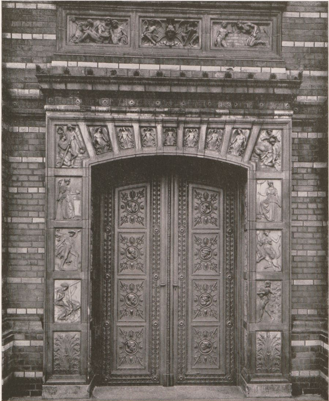
Berlin, Bauakademie. Portal
