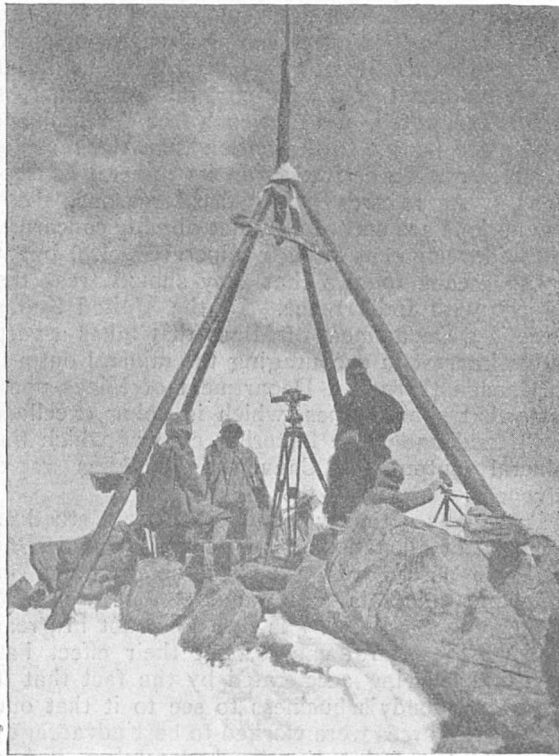
FIG. 1.—On the Russian East Station of Sarblock, 17,284 ft. From "Records of the Survey of India."
