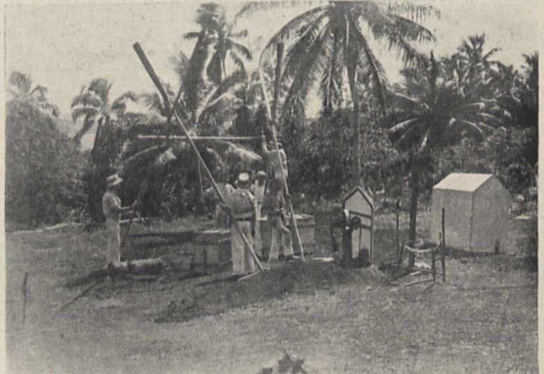
FIG. 4.—The 6-in. prismatic camera in course of erection.
