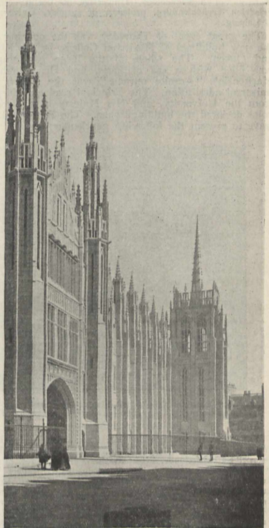
FIG. 2.—Front of Marischal College Buildings, looking southward.
