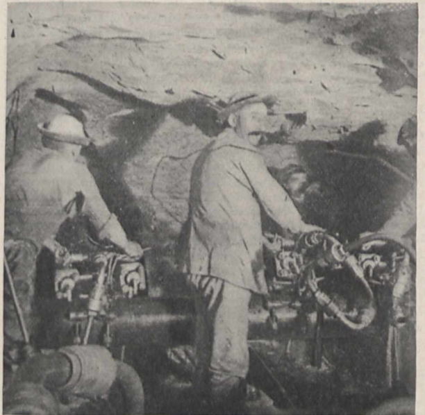
FIG. 2.—The Brandt drill at work at the "face." Daily progress 18 feet. Size of heading 10 feet x 6 feet.
