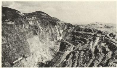
A. RIO TINTO, CORTA DEL SUR, FROM THE WEST-SOUTHWEST. Compare with figure 108. The wall on the left is quartz porphyry, covered with red gossan crust; the terraced slope on the right is black Carboniferous slate dipping steeply north. The cupriferous pyrite lode follows the bottom of the cut and is covered above (in center of photograph) by white clay, produced by the action of H<sub>2</sub>SO<sub>4</sub> on black slate. Photograph by Arnold Heim, February 26, 1932.
