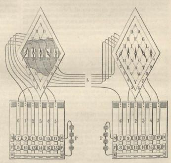
Fig. 26.-Cooke and Wheatstone's five-needle telegraph.]
