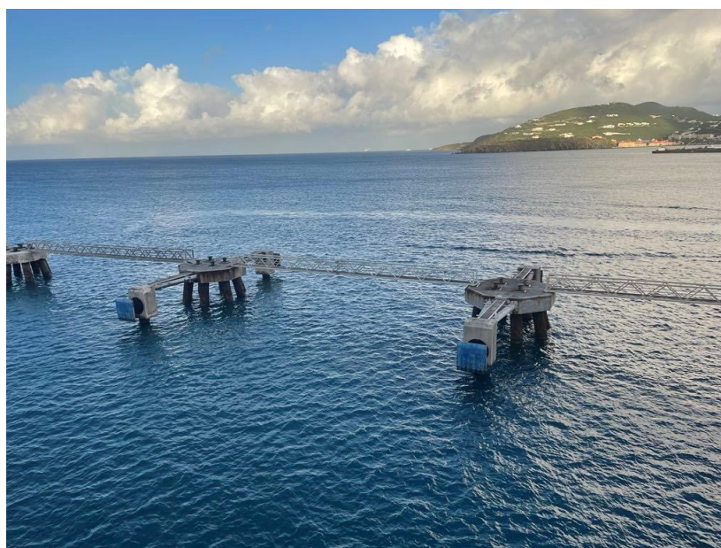
Fig. 2. Example of marine infrastructure – Mooring dolphins and catwalks – Port of St. Maarten /Source: Author's photography/
