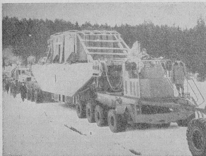
Rys. 17. Transport transformatora na 110 MVA, 380/220/30 kV
