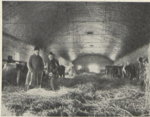
Abb. 93. Innenansicht des Kuhstalls.
