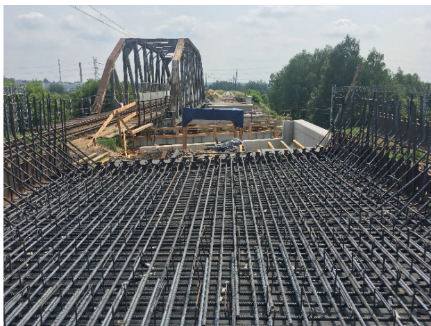
Figure 15: The general view of slab reinforcement.
