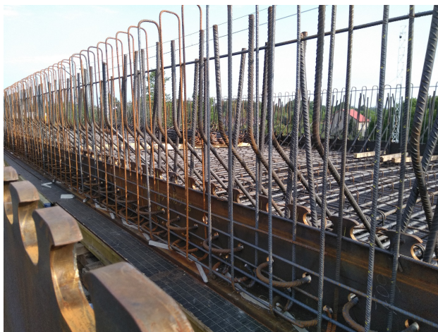
Figure 14: T-sections and reinforcement of bottom part of the superstructure (main stirrups crossing concrete dowels are still missing at this stage, compare Fig. 9).
