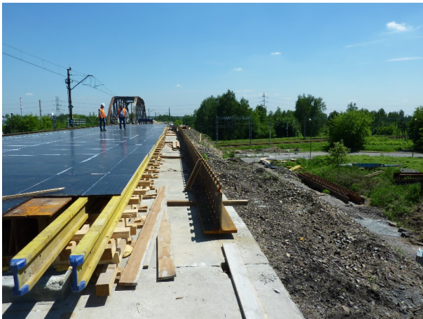
Figure 11: Steel T-sections on site next to scaffolding prepared for in situ slab (picture by Nowak Mosty).
