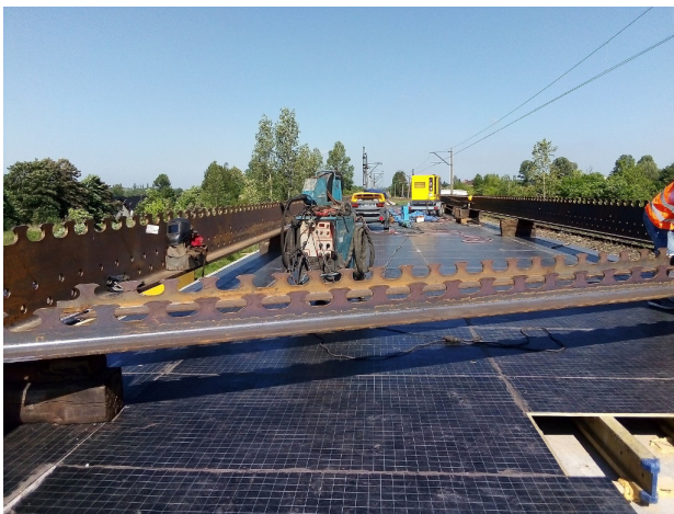
Figure 12: Steel structure after welding (picture by Nowak Mosty): main elements and transversal elements at the edge of slab.
