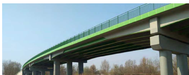
Figure 2: Bridge in Elbląg using both steel and concrete webs in the girder [4, 5].
