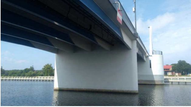
Figure 5: Hybrid beams of Sobieszewo bridge [4, 6].
