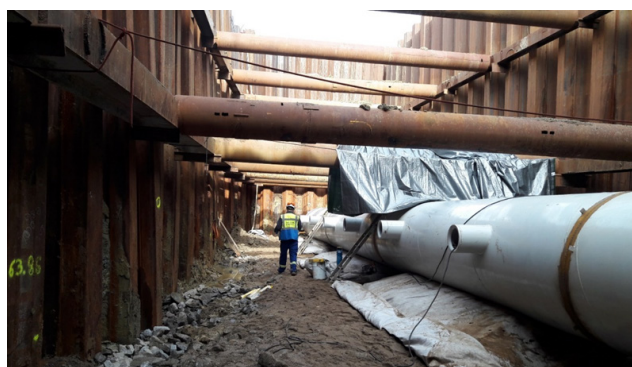
Figure 3: The discharge system during construction.
