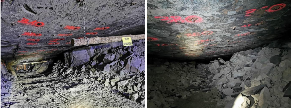
Fig. 6. The test site located in the G-7 department: on the left – just after installation, on the right – after the the high-energy tremor (own compilation)
