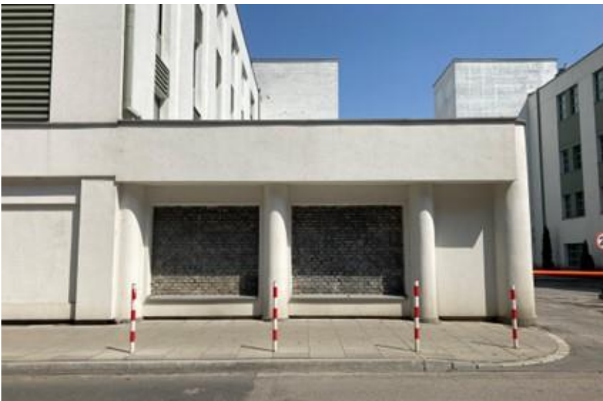
Fig. 6. View of the only authentic fragment of the grey cement brick wall at the entrance gate to the premises of the former K. Szpotkański factory complex. Photo: K. Szuminski, June 2021
