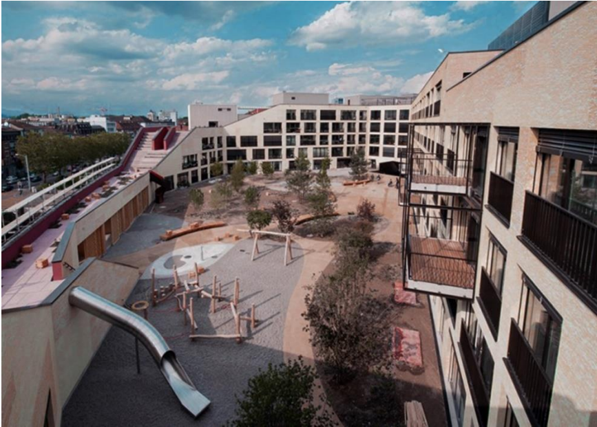
Fig. 4. View towards the inner courtyard of the Kalkbreite building in Zurich.
