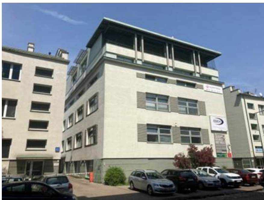
Fig. 2. The plastered facade of factory buildings from the side of Kamionkowska Street. The buildings have lost their original brick character. The authenticity of the former function has been lost. Photo: K. Szumiński, June 2021
