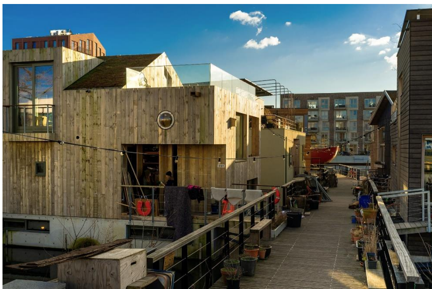
Fig. 2. View towards the floating jetties between the houses in the Schoonschip neighbourhood in Amsterdam. Photo: Agnieszka Kurowska
