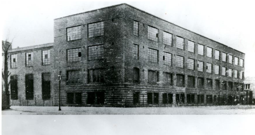
Fig. 4. View of the buildings of the K. Szpotański factory along ul. Kałuszyńska in 1937. Neg. PKZ No. 153949. Source: E. Pustola-Kozłowska, Map of industrial construction in Warsaw, Catalog Volume I, Warsaw 1983
