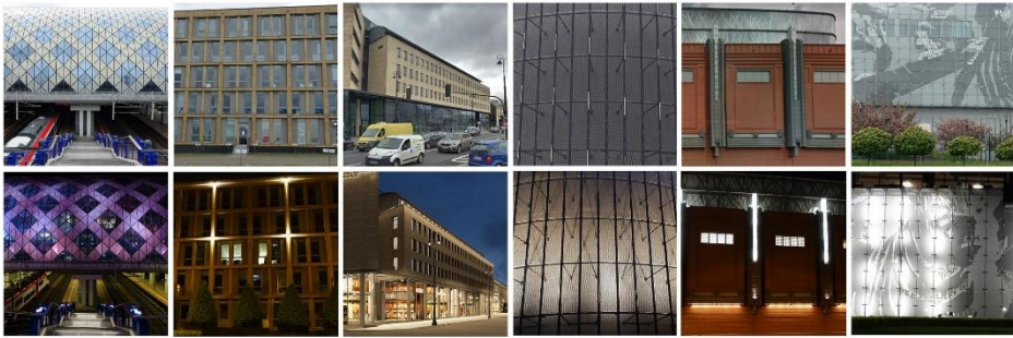
Fig. 6. Examples of buildings with daylight and artificial light together with the applied illumination method. From the left: PKP train station, Poznań PL (flood method); Malta Office Park, Poznań PL (point method); ETHOS office block, Warsaw PL (linear method); Posnania Shopping centre, Poznań PL (mixed method); Sary Browar, Poznań PL (direct method); Malta Shopping centre, Poznań PL (modular method). Photographs by P. Ratajkiewicz, STUDIO DL
