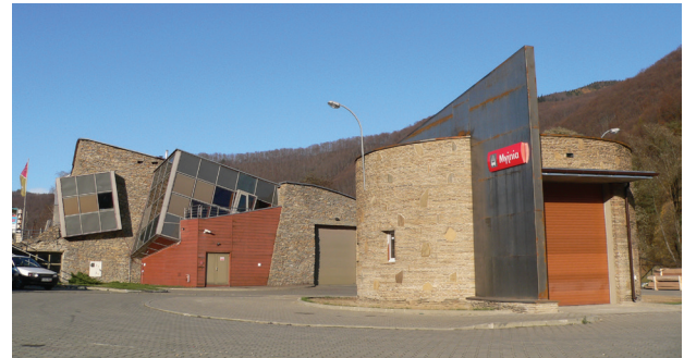
Fig. 2. AL-PLAST service company in Rytrze – view from the south-west (photo by J. Potoczek)
