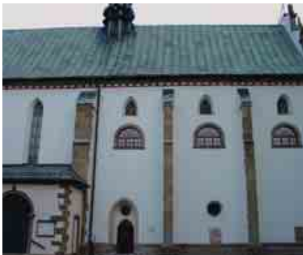
Fig. 15. The view of the north elevation of the monastery's church of Holy Trinity (photo: O.M. Przybyłowicz)
