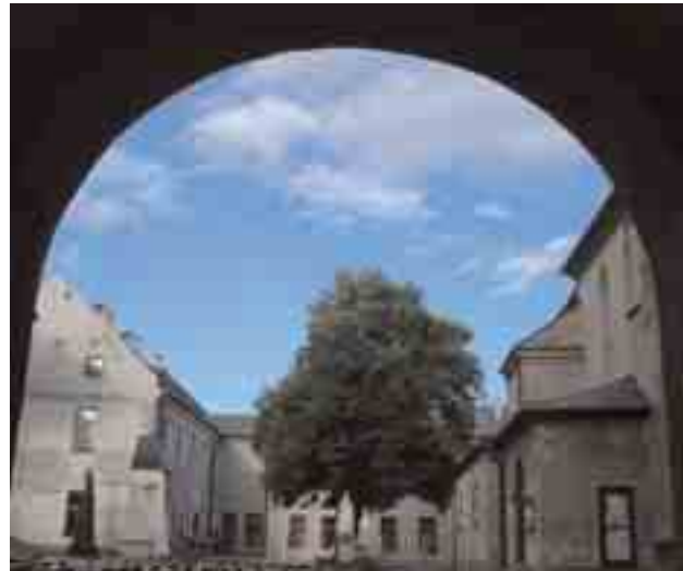
Fig. 12. Interior, north viridarium with the chapelain's house of the 1. half of 17 th c. on the left side and part of the monastic church with the sacristy on the right (photo: O.M. Przybyłowicz)
