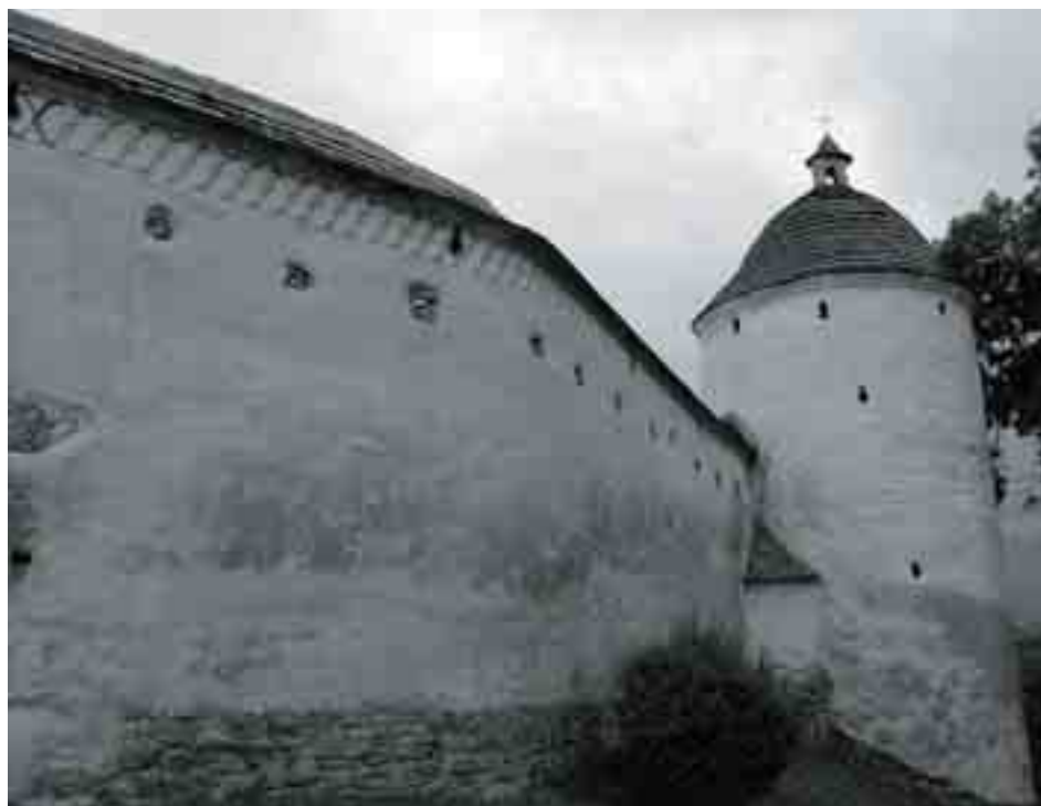
Fig. 7. The south part of cloister walls (16/17 th c.) with a tower under the modern plaster before preservation in 2008 (photo: O.M. Przybyłowicz)
