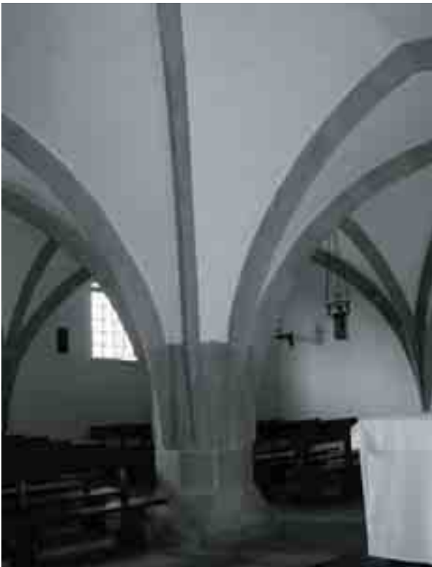
Fig. 3. The old monastic chapter house of 13/14 th c. with main column, cantilever and leading out of the ribs (photo: O.M. Przybyłowicz)
