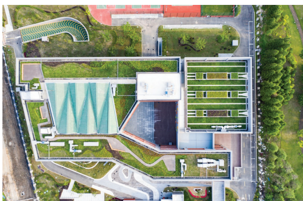
Fig. 6. Rooftop Gardens Shanghai Thomas School, Shanghai (project by Architects TJAD, photo by Youn Ma, 2019, source: [34])
