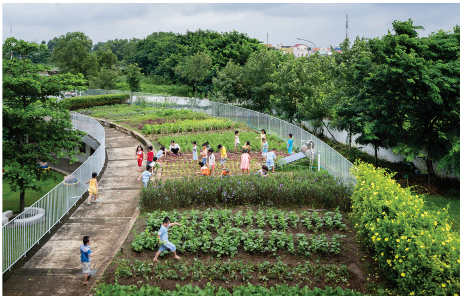
Fig. 11. Vegetable gardens on the roof of the kindergarten in Bien Hoa (Vietnam) (project by VTN Architects, photo by Gremesy, Hiroyuki Oki, 2013, source: [41])
