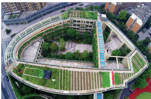
Fig. 5. The roof garden of the elementary school at Puijia in Shanghai (project by Li Bojun with the team, 2015, photo by an unknown author, source: [33])
