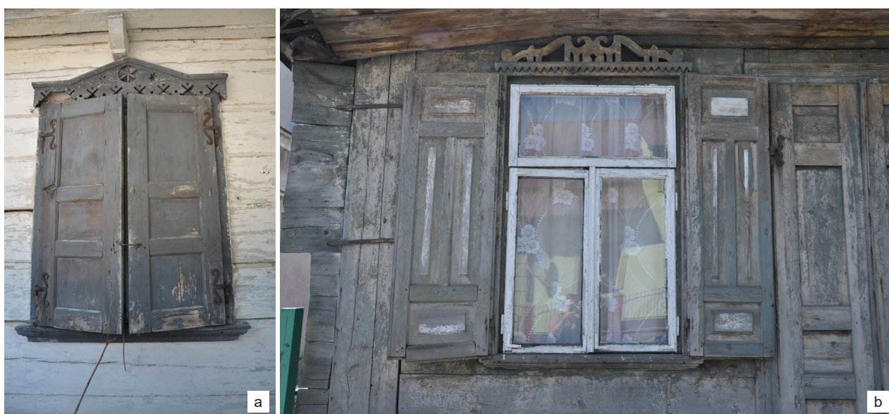
Fig. 10. A window frame with a decorative window drip and shutters in a one-story single-family house:
