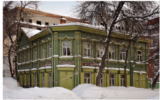
Fig. 1. An example of traditional Russian wooden buildings in Samara (photo by E. Pol, 2011)
