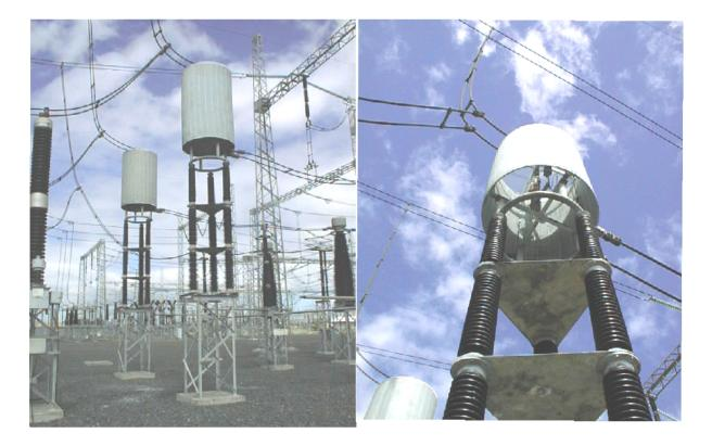
Fig. 1.24: Typical Line Traps
