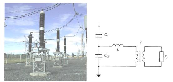
Fig. 1.22 : A high voltage Capacitive Voltage Transformer(CVT)
