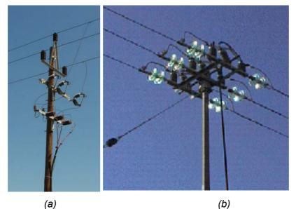
Fig. 1.30: (a) Cut-out (drop-out) Fuse assembly (b) Isolator (link) assembly
