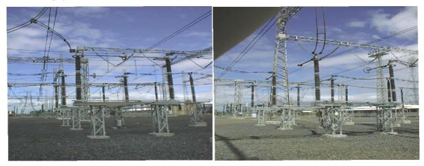
(a) (b) Fig. 1.31: Typical rotating arm isolators: (a) Isolator closed and (b) Isolator open.
