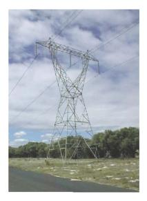
Fig. 5.16: High voltage line with two overhead screen wires
