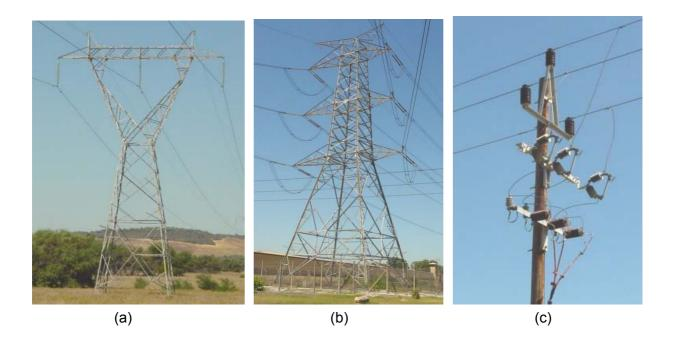
Fig. 1.9: Typical overhead high voltage lines: (a): 400 kV suspension tower, (b) 400 kV double circuit strain tower and (c) 22 kV woodpole distribution line with fused cable connection.
