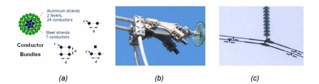
Fig. 1.11: Examples of conductor power line components: (a) Detail of ACSR conductor,(b) Pistol grip connection of a conductor to a strain insulator and (c) Wind vibration dampers.
